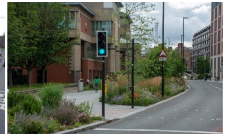
Example of rain gardens used to reduce hard landscaping
