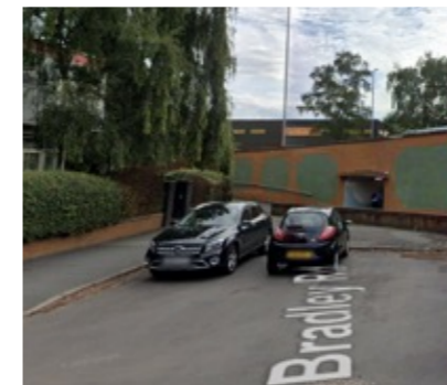
Current Bradley Road subway entrance
