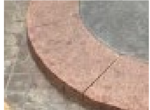
RED GRANITE KERB to pavement edge
