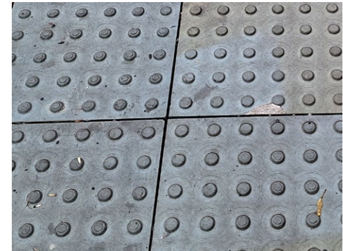
YORKSTONE BLISTER PAVING for uncontrolled crossing points
