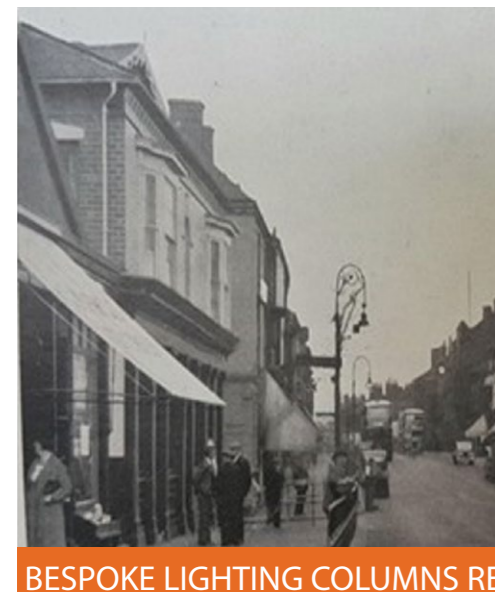
BESPOKE LIGHTING COLUMNS RESTORED
